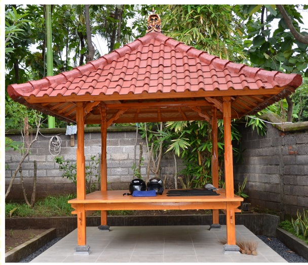
Figure 4. Scaled timber framed pavilion "Bale" type structure for Gazebo.
