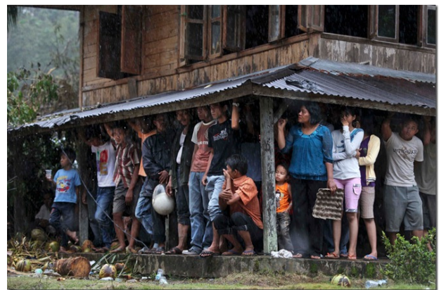
Figure 1. Buildings in Padang, Indonesia after the September 30, 2009 earthquake (7.6 on Richter scale). A two-storey timber framed residential building providing safe shelter from rain after the earthquake. [Photo by Kevin Frayer, reproduced by permission ( Frayer 2009 )]
