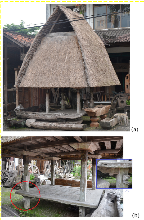
Figure 2. Typical barn “Jineng” in Bali-Indonesia. (a). Front view of timber-framed barn. (b). Close up of the platform of the barn.
